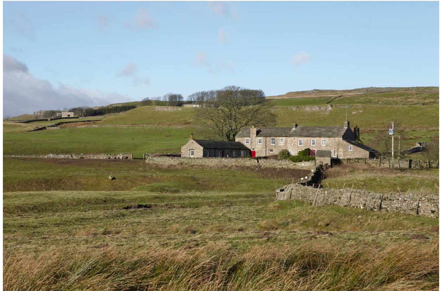
Borrowdale House, Kitty's Barn and Borrowdale Cottage North Stainmore, Kirkby Stephen, Cumbria, CA17 4DZ
